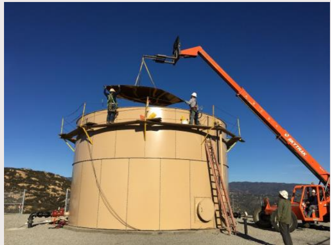
Finishing touches on the water tower.
