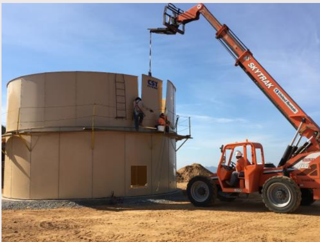
Crews building the water tower.
